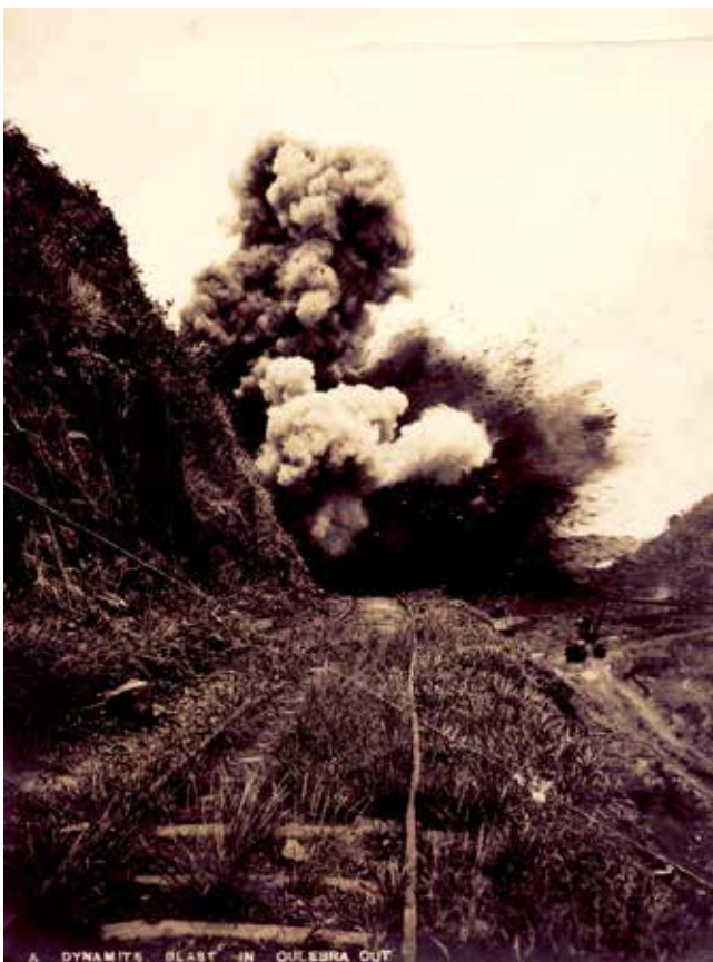
Dynamite blast during excavation of Panama Canal, ca 1904–1914 Digital Library of the Caribbean
